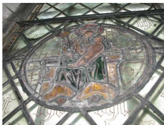
External glazing visible through internal panel.
